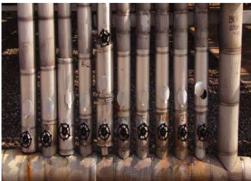
Piping & Field Insulation
